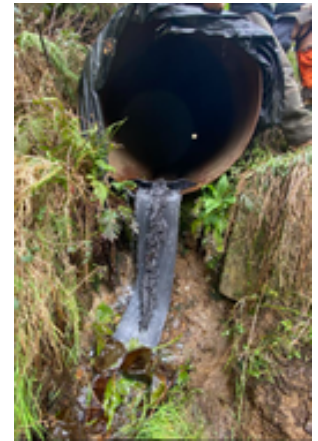
EXAMPLE OF BEFORE AND AFTER OF CULVERT REMEDIATION – WITH BAFFLES, MUSSEL ROPE & RAMP
